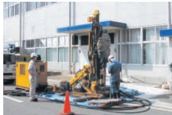
Soil Bore-hole Survey at Tatsuno Site
