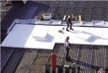
Photo 5 OWI has installed heat insulation in the roof of its plant.
